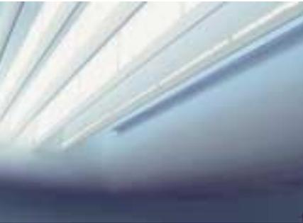
When white single-ply roofing (see previous page) is placed directly in front of the south-facing roof monitors, the glazing area in the monitors is able to be reduced by up to 20% because of the additional reflected radiation entering the monitor.
